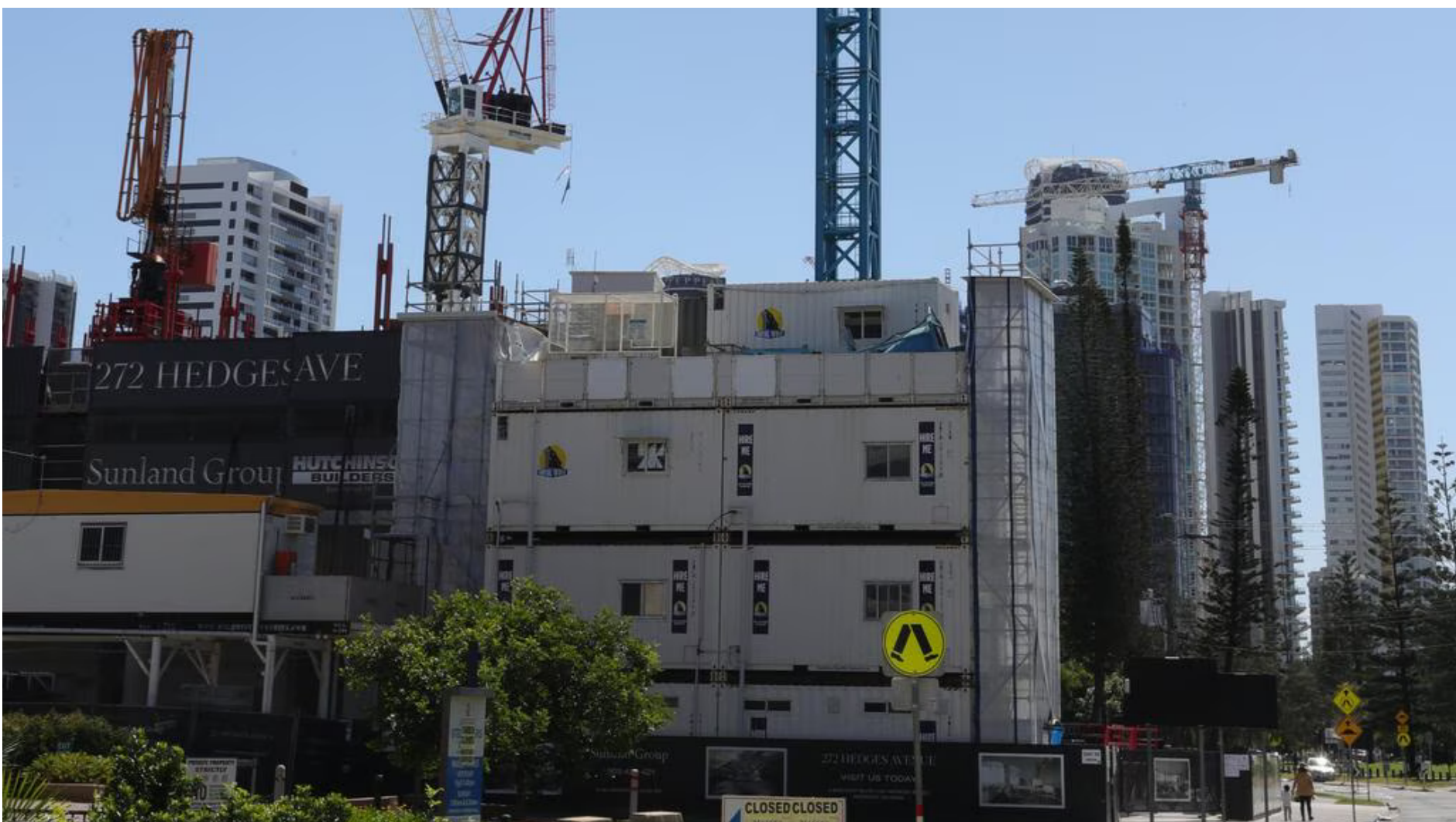
Construction work on the Gold Coast on new towers. Picture: Glenn Hampson.
